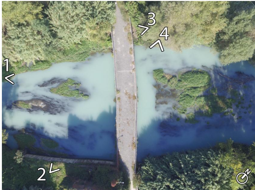
Figure 10. Location of the cones of vision used in thermographic investigations.
