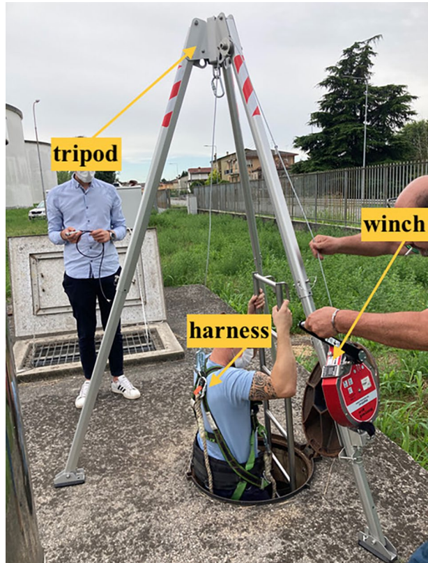
Fig. 1 A fall-arrest and rescue system for emergency retrieval, in a confined space, as prescribed by law in Italy
