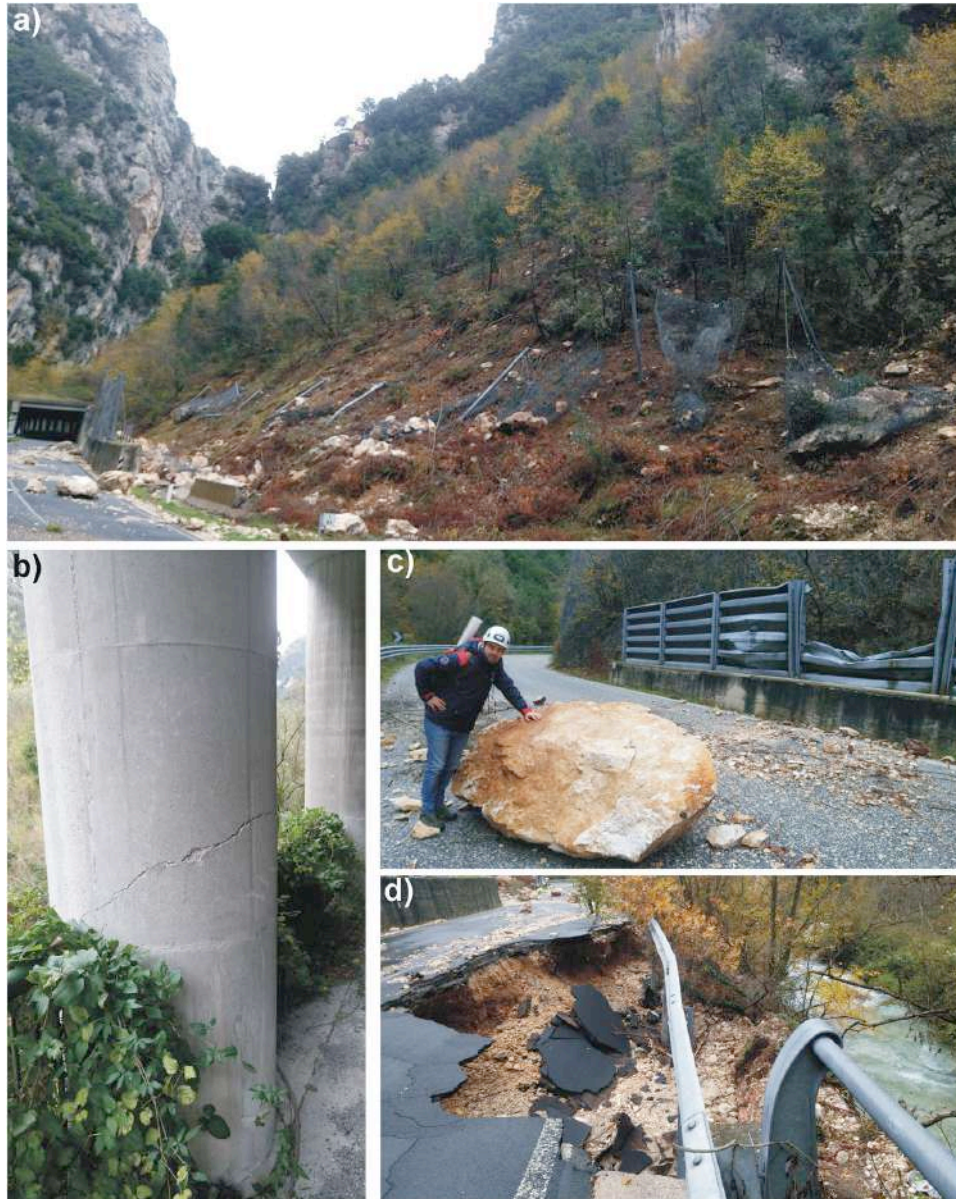
367 Figure 4 Damages to infrastructures induced by seismic activity and related rockfalls within the study area. a) 368 overturning and displacement of elastic nets (point g in Fig. 3); b) pillar breaking and distortion of a rockfall 369 protection tunnel (point i in Fig. 3); c) breaking of rigid barriers by a rock block (point d in Fig. 3); d) erosion of 370 road embankment (point i in Fig. 3) by water flow related to landslide dam (point o in Fig. 3).
