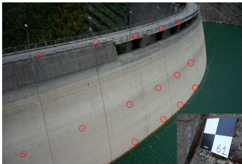
Figure 3. Upstream face of the Ridracoli dam. The red circles indicate marker positions. The small panel shows a marker applied on the structure.
