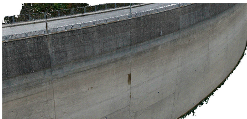
Figure 7. UAV dense 3D point cloud of a portion of the upstream face of the Ridracoli dam.
