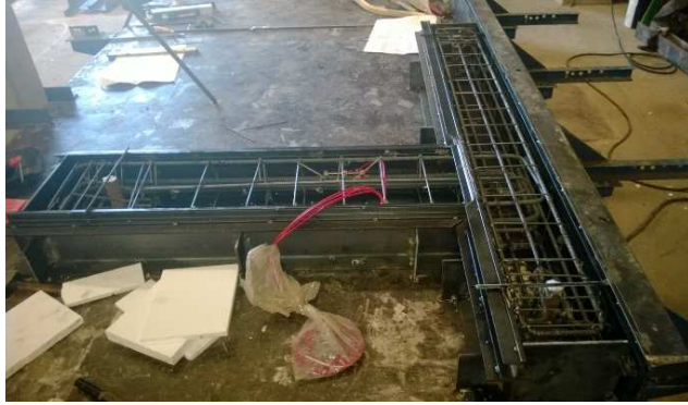
Figure 7: Reinforcement and formwork of the cast-in-situ specimen.
