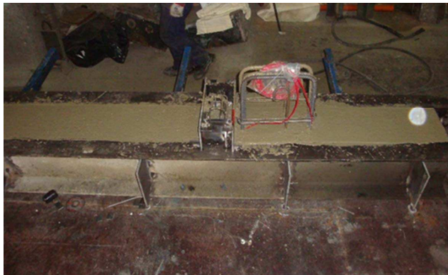
Figure 8: Precast column just after the concreting.
